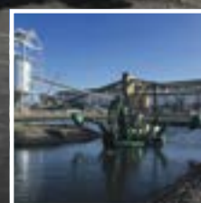
COAL SETTLEMENT POND
