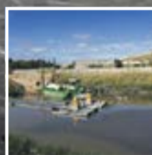
CLEANING A PUMP INLET
