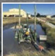
CLEANING A SETTLEMENT POND
